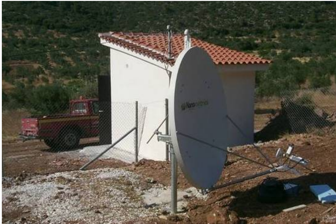
Figure 2. View of Loutraki (LTK) station.
